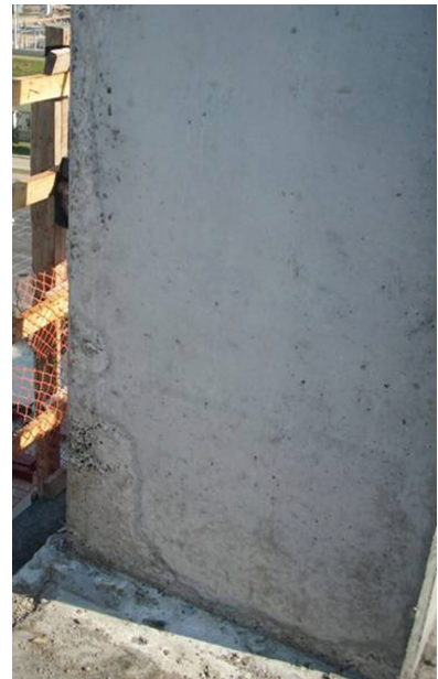
Results from a standard industry vibrator overspeeding
